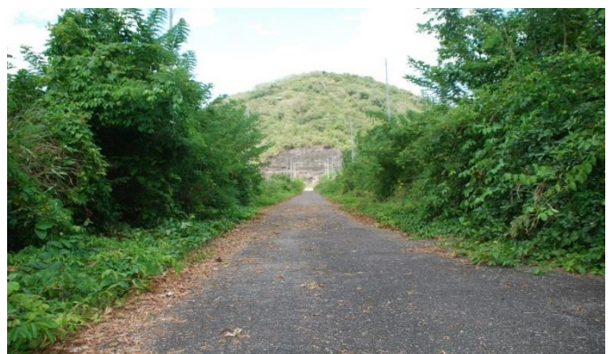
Figura 3: Cresta de la Presa Ing. Francisco C. Amelinck (2017)
